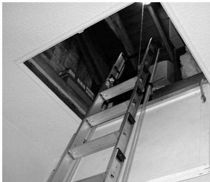
View of access to the attic with the Televator extended.
